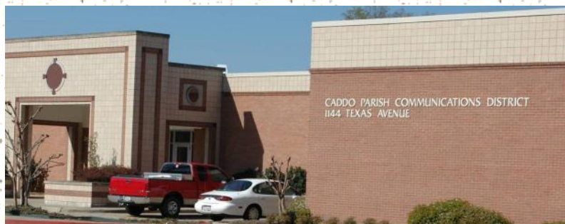
The Joint Communications Center serves the Caddo Sheriff Office, Shreveport Police Department and Shreveport Fire Department
